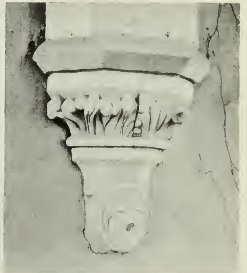
WETHERSFIELD CHURCH. E. respond, S. arcade ; early 14th-century.
